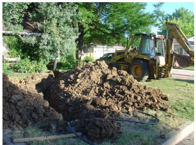
Trenching to add a manifold connecting the two boreholes
