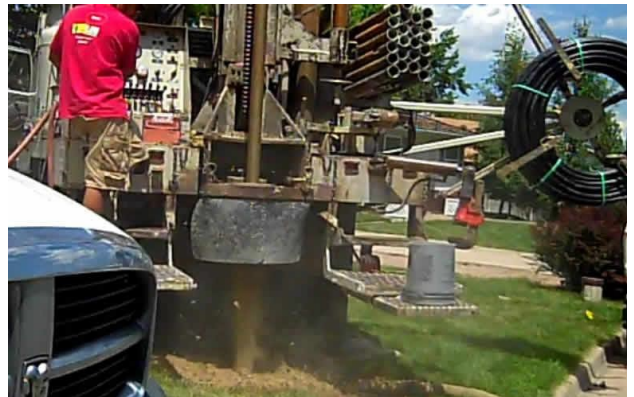
Drilling first 300' deep hole
