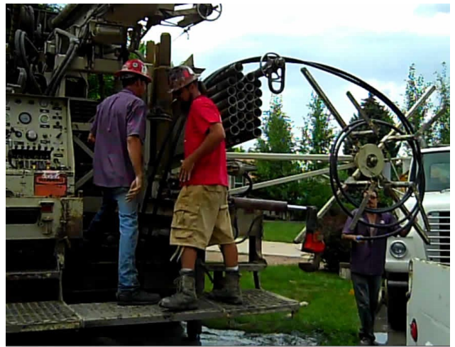
Inserting the U- shaped black plastic tubing 300' down into the borehole
