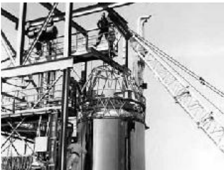
Figure 95 Centaur is raised into the "J" Tower for testing at Point Loma, early 1960s. Credit: Lockheed Martin
