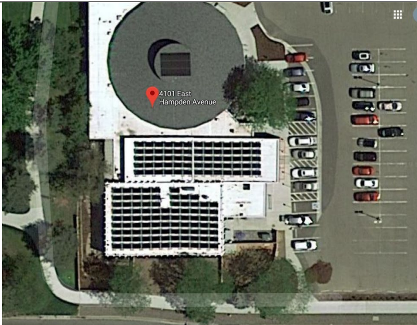
Figure 62 Minimal Shading from Deciduous Trees with Leaves Mid Summer – Local Time ~ 10:00 am.
