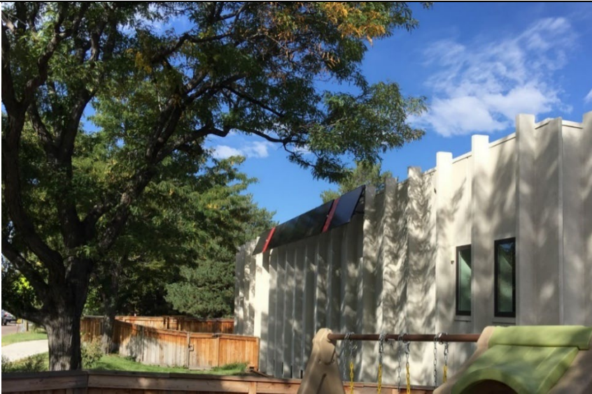
Figure 63 Early Morning Major Shading by Two Deciduous Trees on 6 Awning Modules (with micro inverters). Photo Taken September 16, 2019 at 9:16 Solar Time
