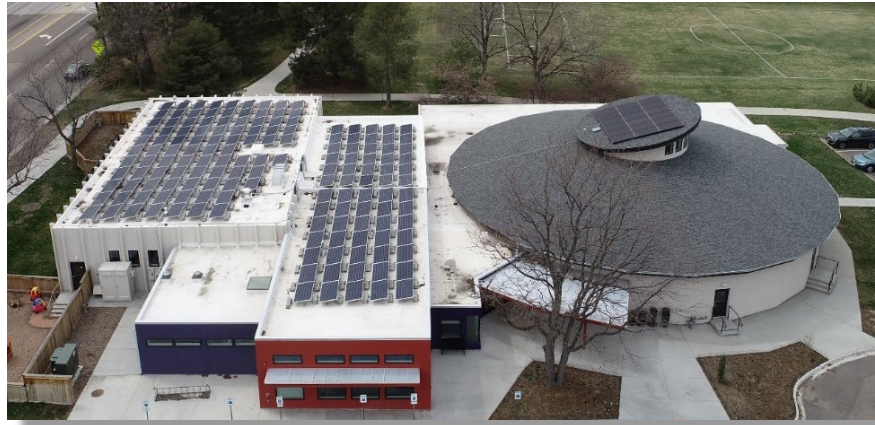
Figure 5 The Sustainable Energy System utilizes a 57 kW solar PV system to generate electric power and a 45 Ton ground-source heat pump system for heating and cooling.
